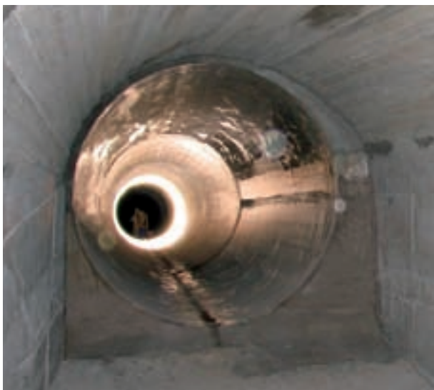
Dual bolt mechanical coupling
